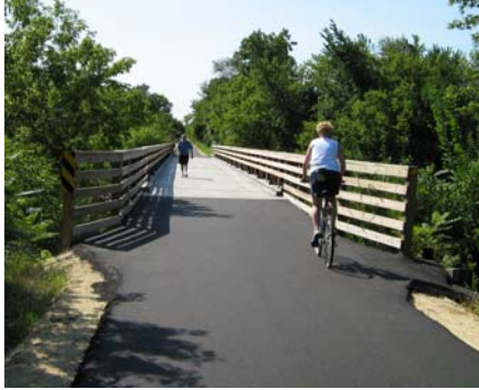
Paved not within road right-of-way
