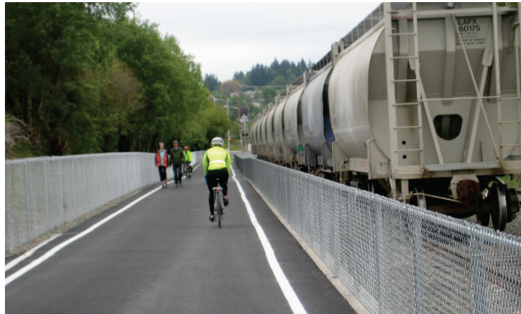
Figure 2-6: A “rail with trail”, or shared use path next to a rail corridor, in Seattle, WA
