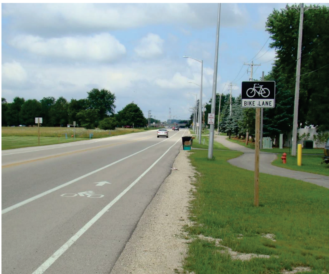
State Highway 60 in the Village of Jackson was rebuilt recently with bike lanes and a sidepath on the north side of the highway.
