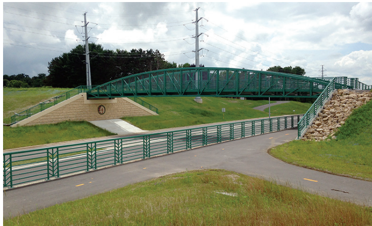
Figure 2-9: A bicycle and pedestrian bridge over CTH PD (McKee Road) in Madison, WI connects the Ice Age Junction Path system
